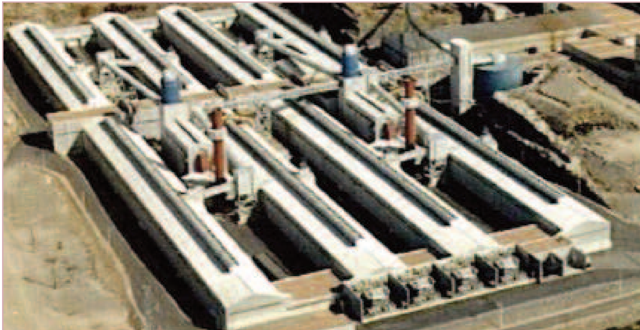
Figure 1. Typical aluminum smelter rooftop configuration. A typical arrangement of ridge vents at an aluminum smelter with an elongated rooftop vent. The buoyancy is related to the elongated internal arrangement of potrooms and other operations. These are both emission and heat emitting.
